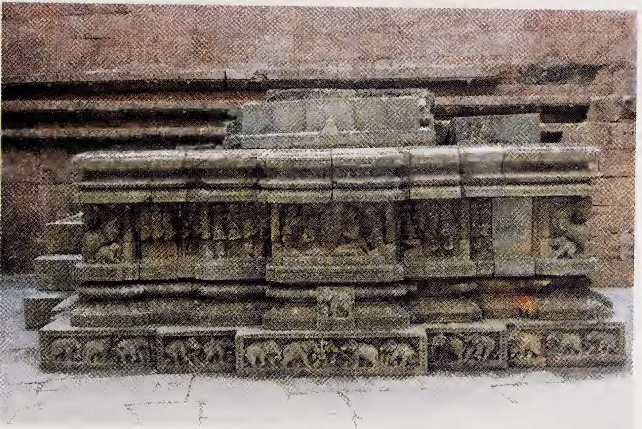
Deula: Platform inside the sanctum view from the East.
